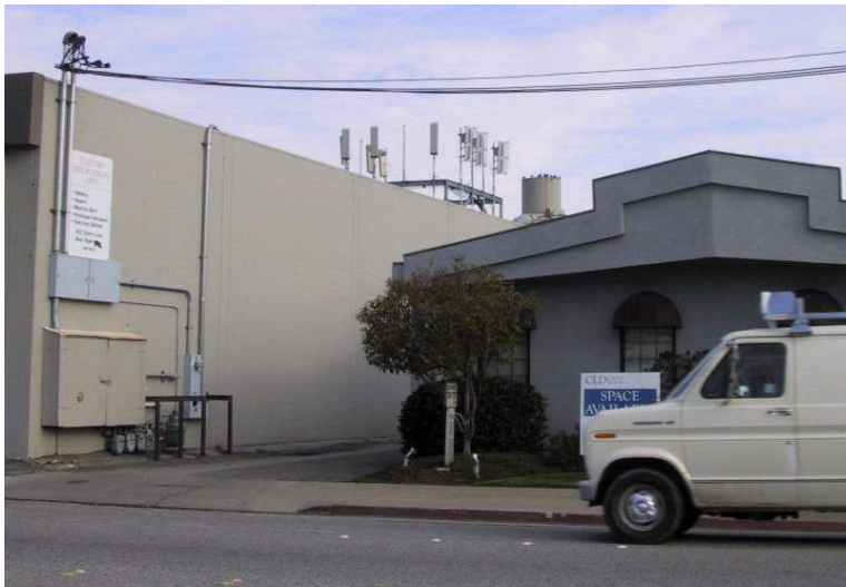
Figure 39 - Adjacent Building. Down Tilt Antennas
