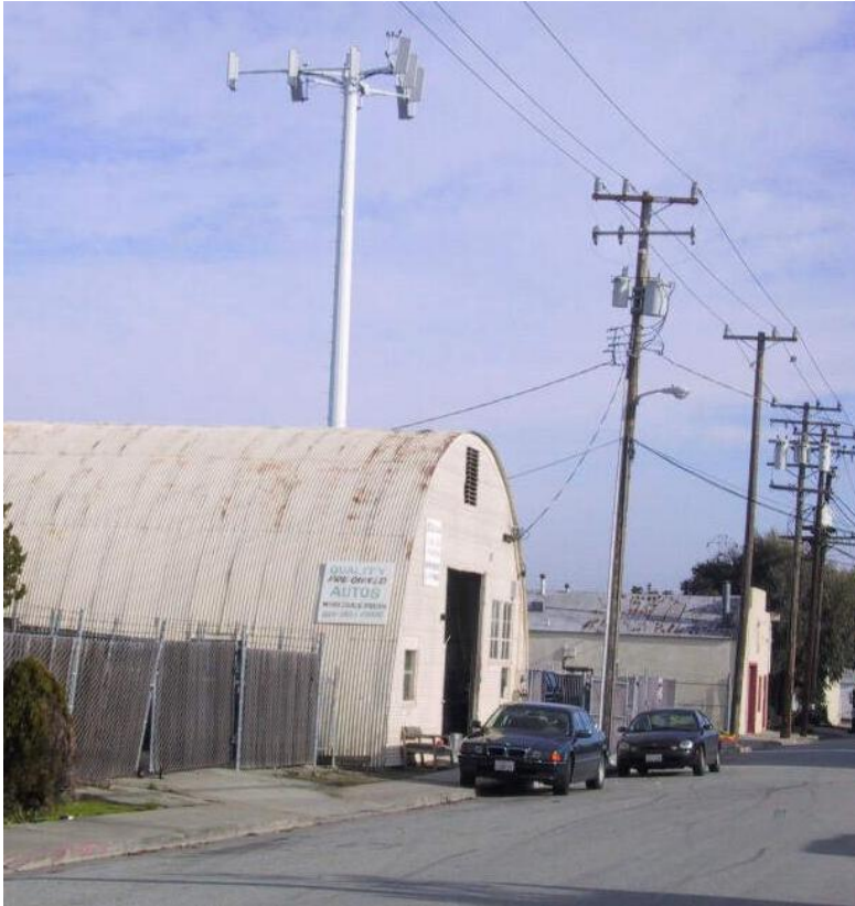
Figure 37 - 40 Ft Tower with Down Tilted Directional Antennas
